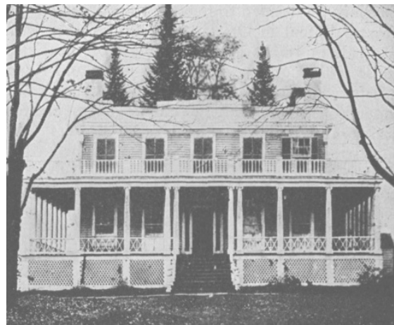
THE HOUSE AT LAKELANDS, as originally built
