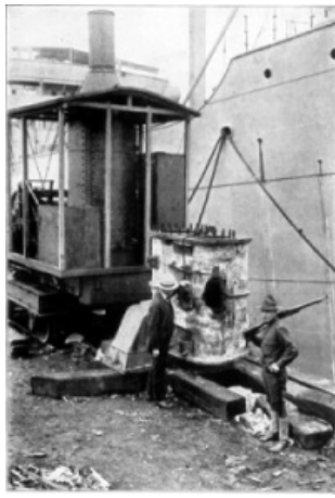
From a photograph copyright by International Film Service. Repairing a damaged cylinder of a German ship for federal service.
