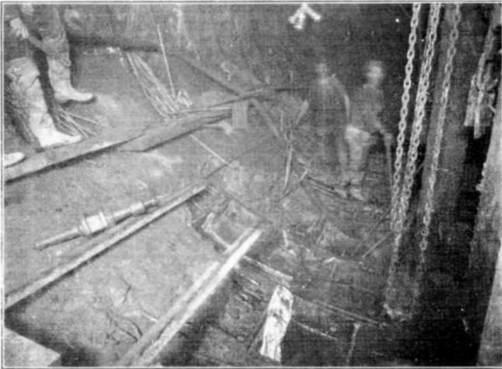
PLATE LXXIII, FIG. 1.—TEMPORARY REINFORCEMENT OF BROKEN PLATES AND REMOVAL OF A PLATE IN SECTIONS.
