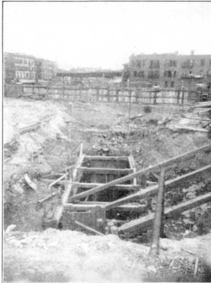
PLATE LXX, FIG. 1.—SMALL SHAFT SUNK TO ROCK.
