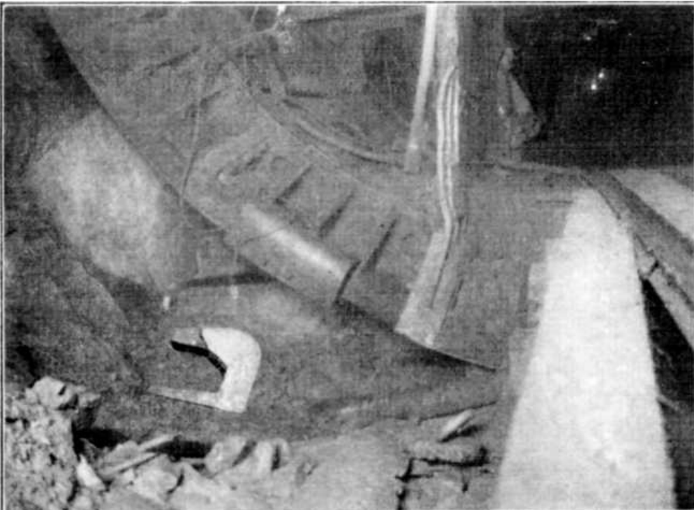
PLATE LXXIII, FIG. 2.—HEAVY CAST-STEEL PATCH ATTACHED TO BENT SEGMENT OF CUTTING EDGE.
