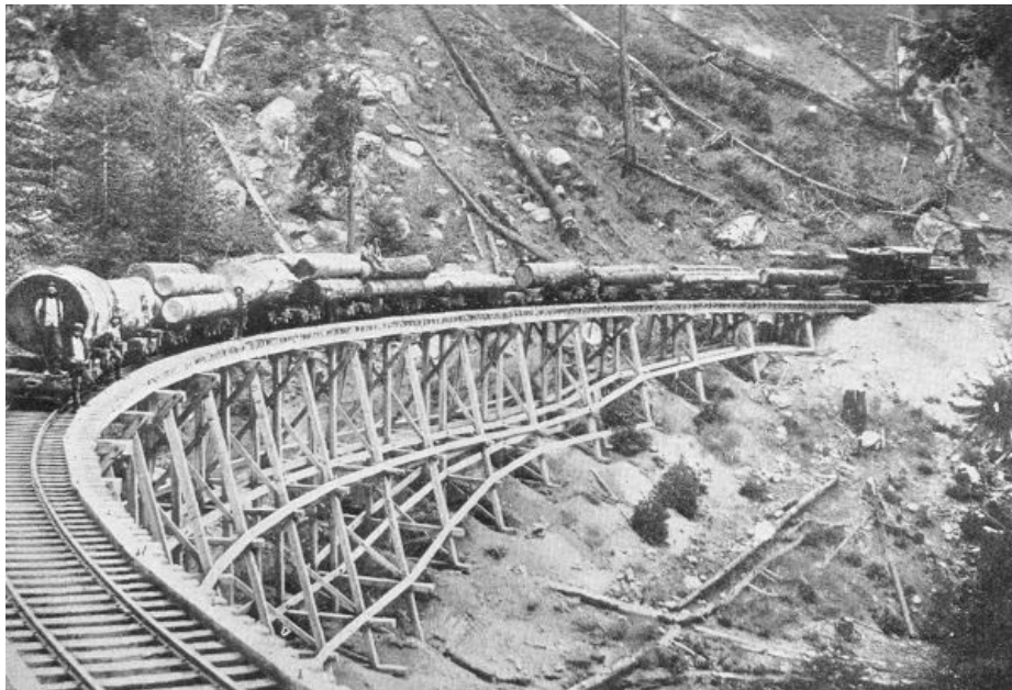
TRAIN-LOAD FROM ONE TREE. Temporary railroad built through the forest to the sawmill. Photograph by U. S. Forest Service.
