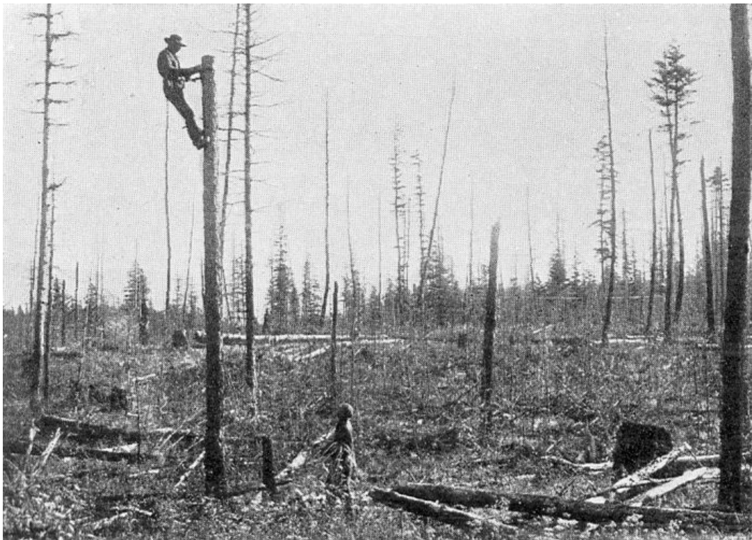
RUNNING A TELEPHONE LINK.
