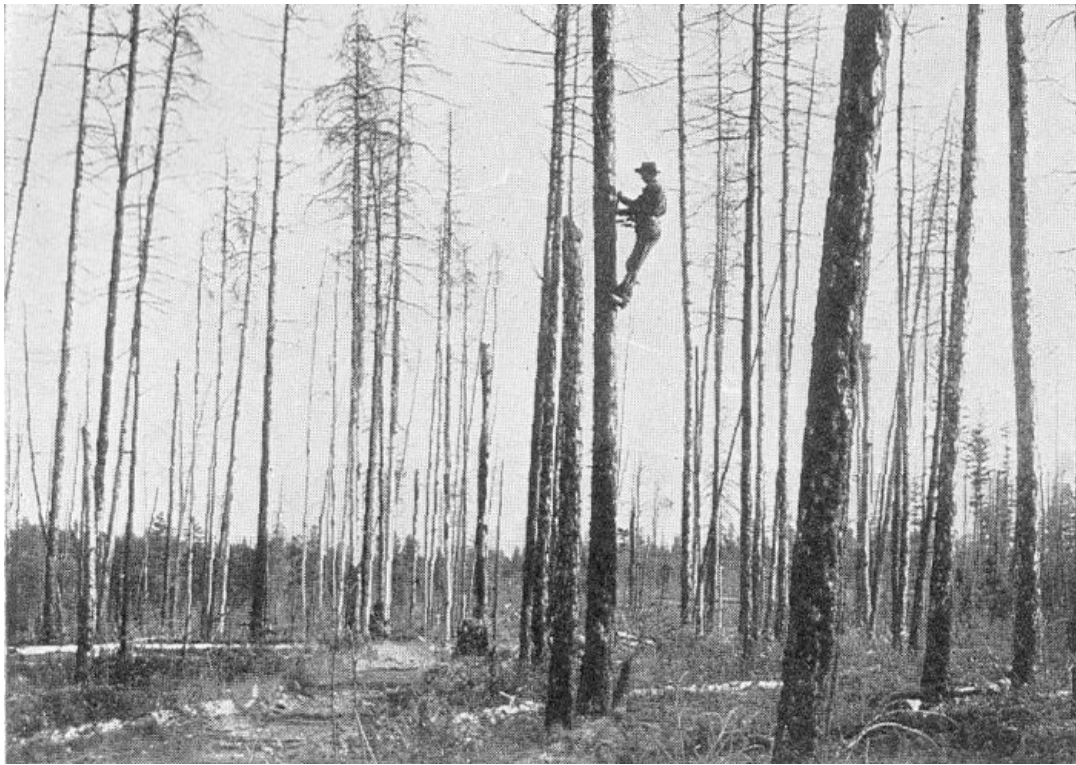
RUNNING A TELEPHONE LINK.
