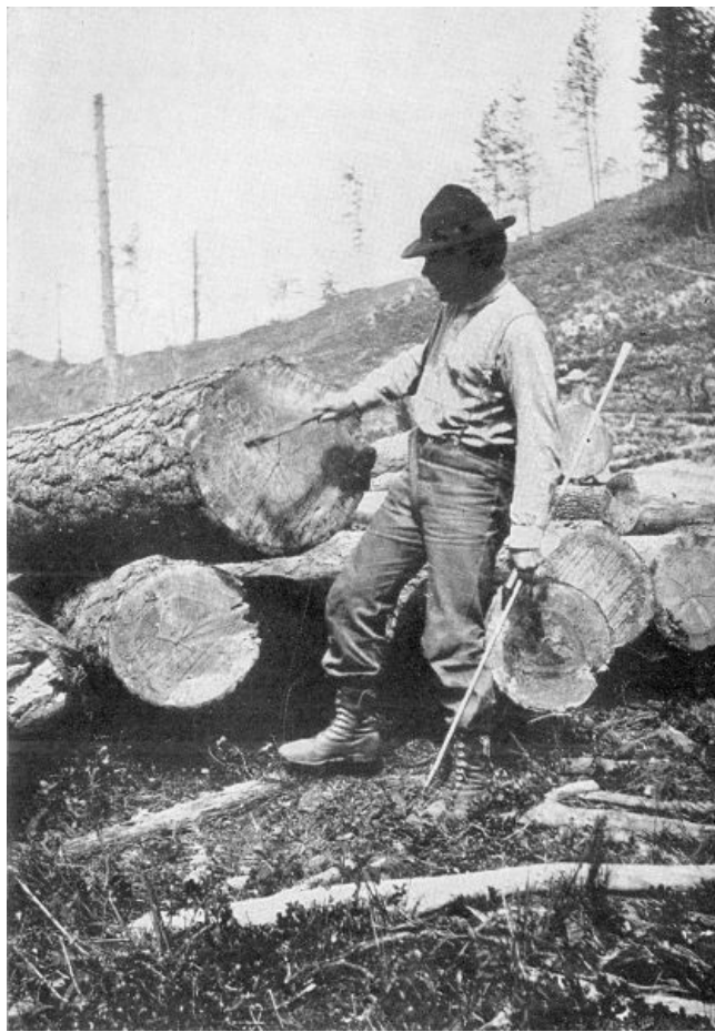
STAMPING IT GOVERNMENT PROPERTY. McGinnis marking "U. S." on timber that has been scaled and measured up. Photograph by U. S. Forest Service.
