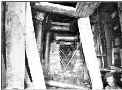
PLATE LIX, FIG. 4.—TIMBERING AND RUBBLE MASONRY OVER I-BEAMS.
