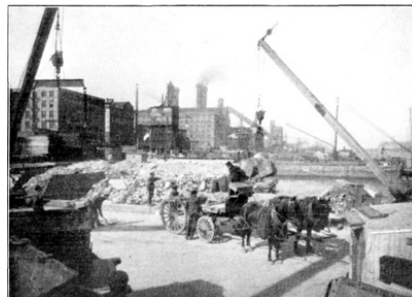
PLATE LVIII, FIG. 4.—LOADING SPOIL ON BARGES, 35TH STREET PIER.
