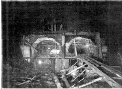
PLATE LIX, FIG. 3.—FIRST SECTION OF CONCRETE LINING AT FIFTH AVENUE.
