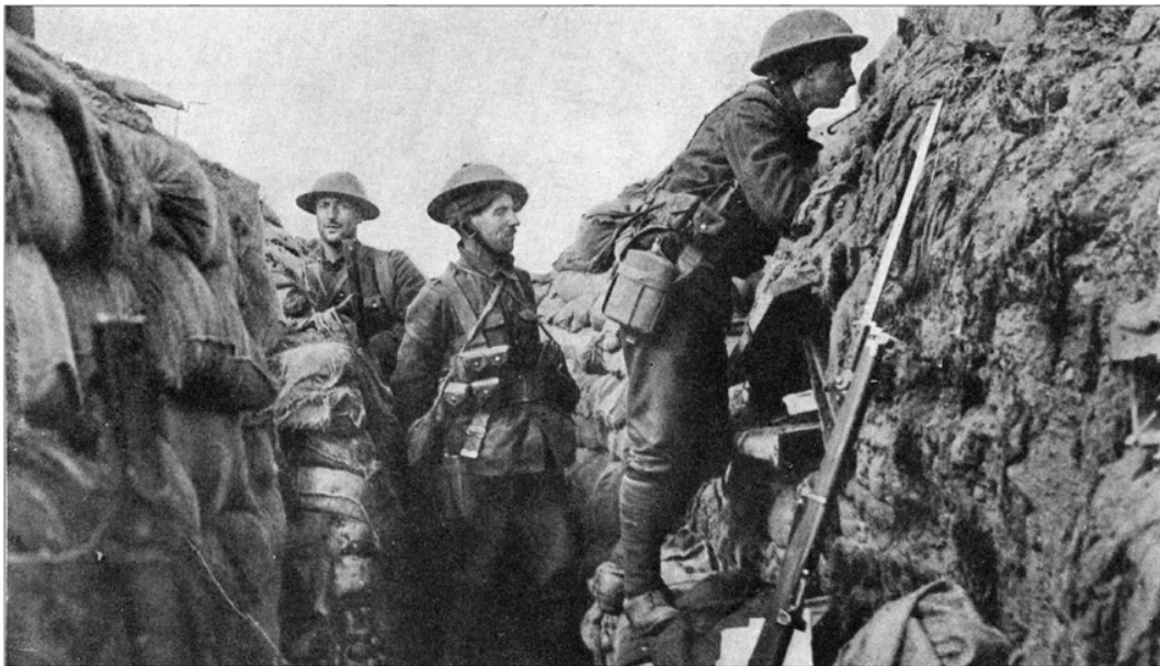
The Fire Trench.
