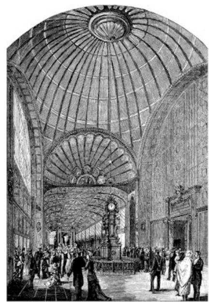
GRAND CUPOLA AT ONE OF THE CHIEF ENTRANCES TO THE MAIN BUILDING.
