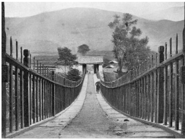
INSIDE VIEW OF A SUSPENSION BRIDGE IN FAR WESTERN CHINA.
