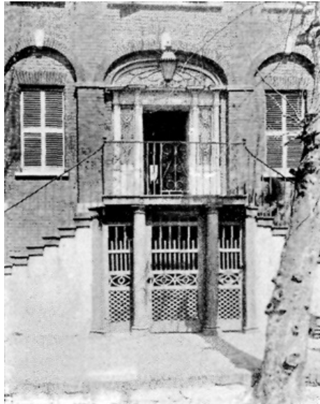
Doorway to the Bull House, Charleston.
