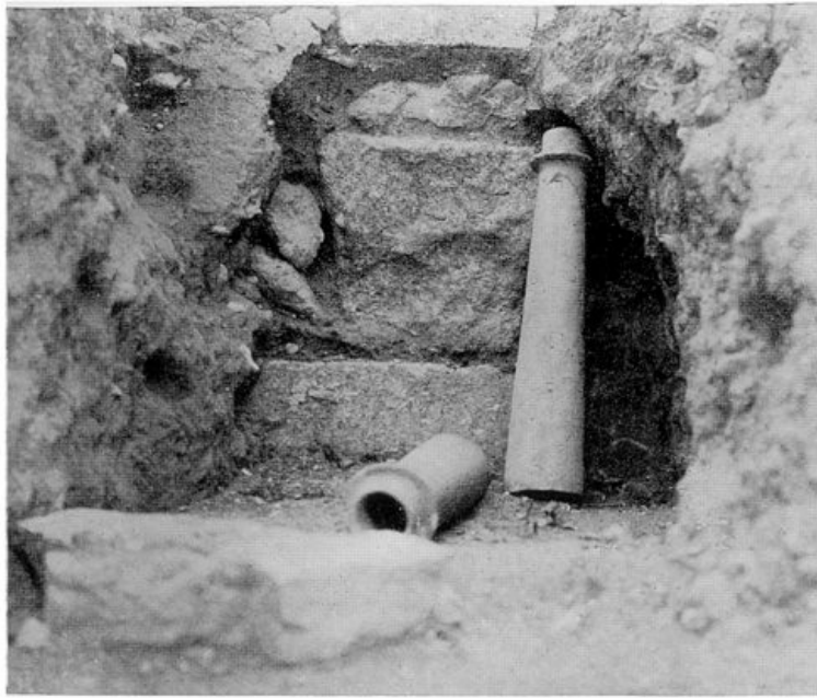
(2) TERRA-COTTA DRAIN PIPES (p. 98)
