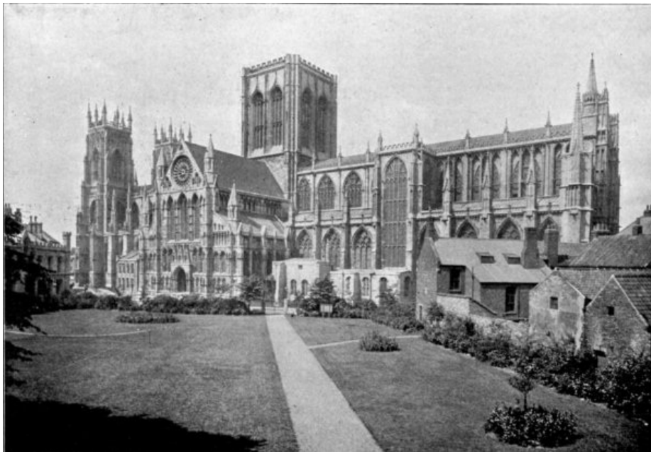
The Exterior, from the South-East.
