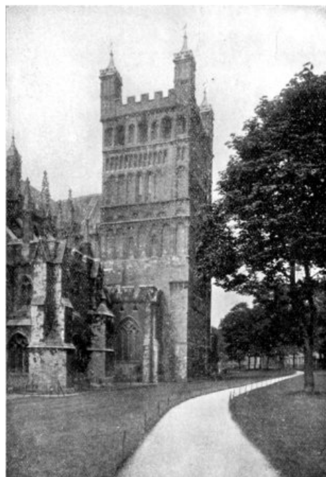
THE NORTHERN TOWER.
