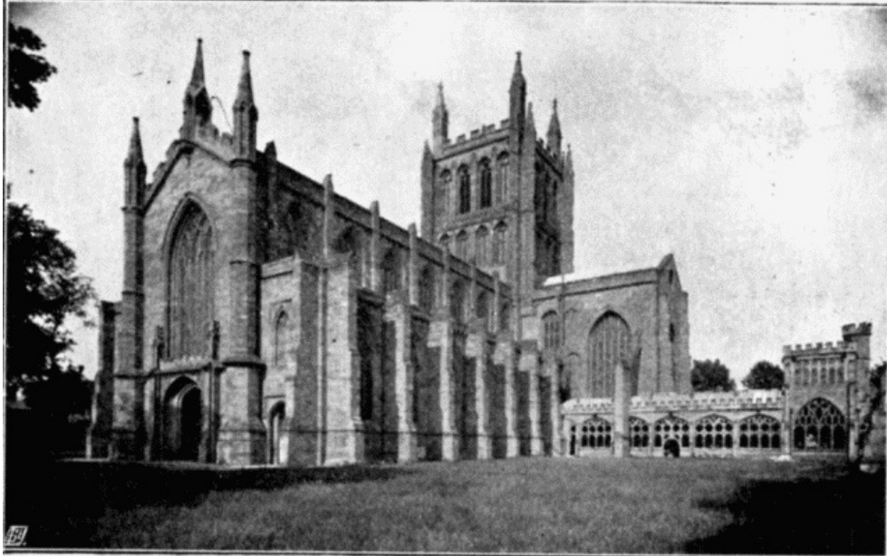
GENERAL VIEW, FROM THE WEST.
