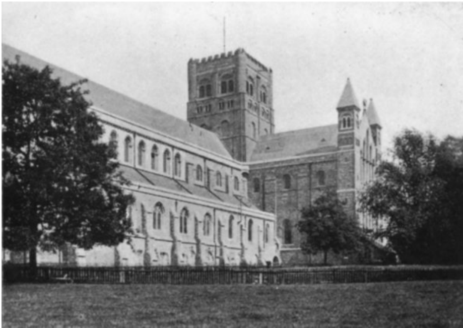
THE SOUTH TRANSEPT AS REBUILT.
