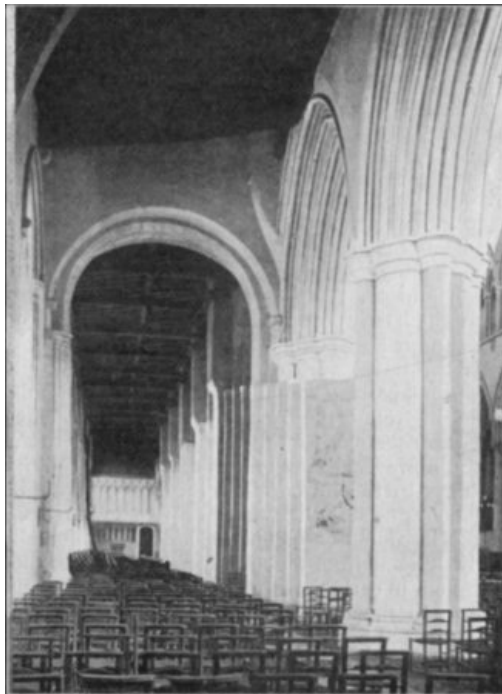
NORTH AISLE OF NAVE.
