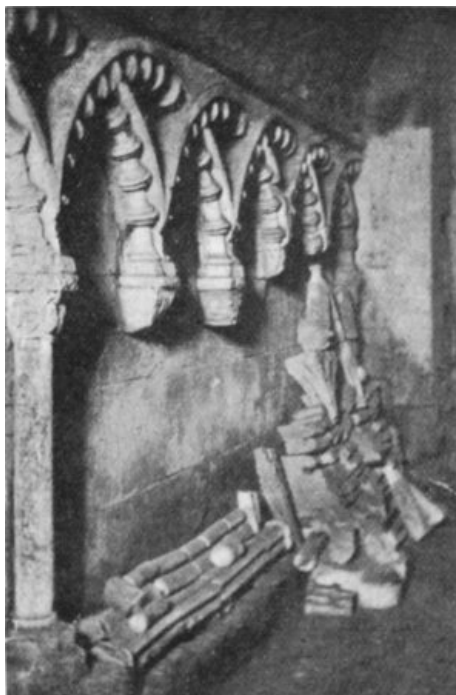
THE ARCADE IN THE SLYPE BEFORE ITS REMOVAL.
