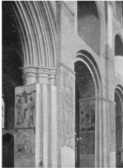
ARCADE ON NORTH SIDE OF NAVE.
