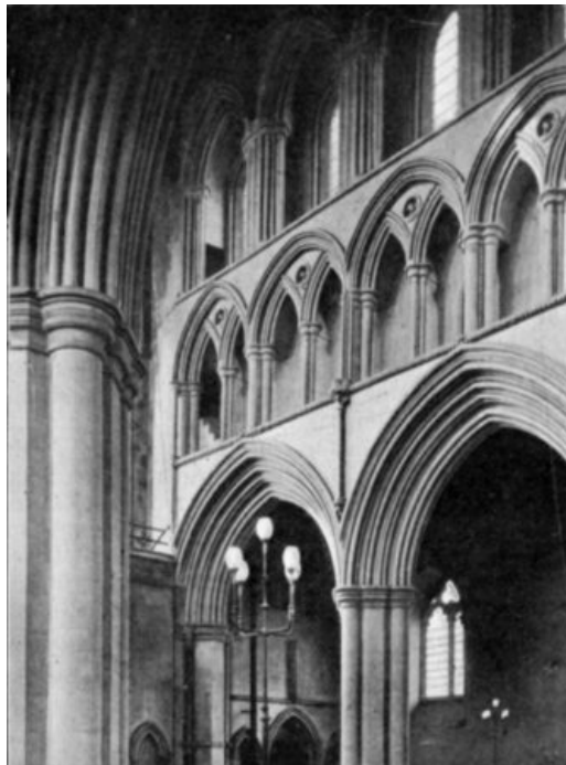
NORTH NAVE ARCADE: WESTERN END.
