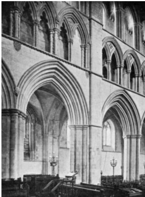
SOUTH NAVE ARCADE, SHOWING THE JUNCTION OF THIRTEENTH AND FOURTEENTH-CENTURY WORK.
