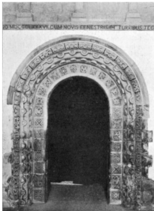
DOORWAY IN SOUTH TRANSEPT.
