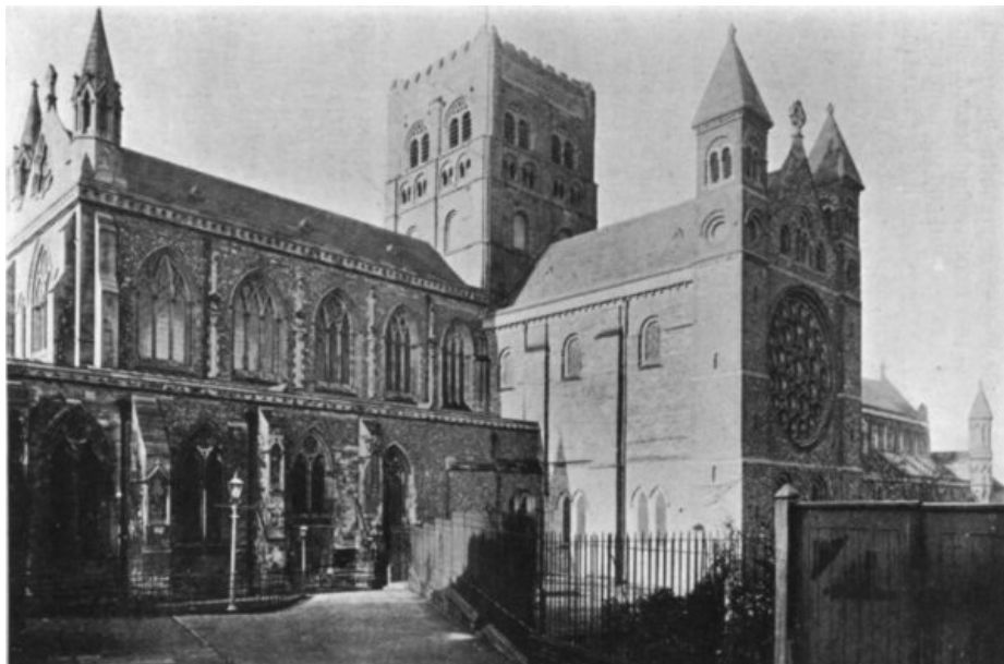
THE CATHEDRAL FROM THE NORTH-EAST.
