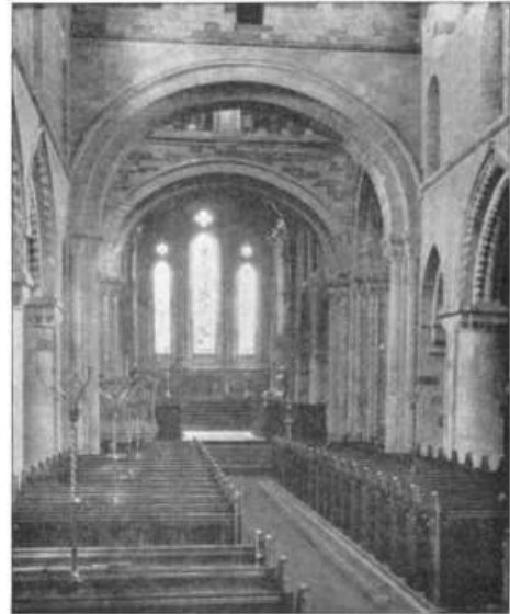
THE TOWER ARCHES.
