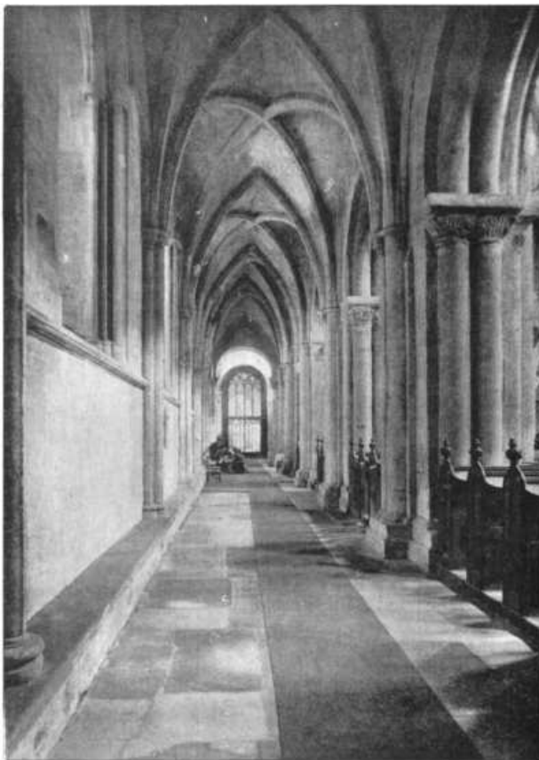
THE NORTH AISLE OF NAVE.
