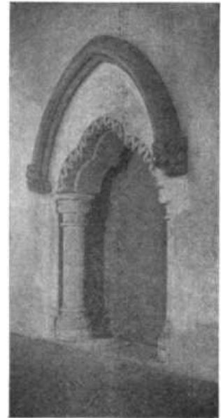
THIRTEENTH-CENTURY PISCINA IN SOUTH TRANSEPT.
