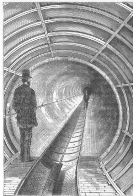
TUNNEL UNDER BROADWAY.
