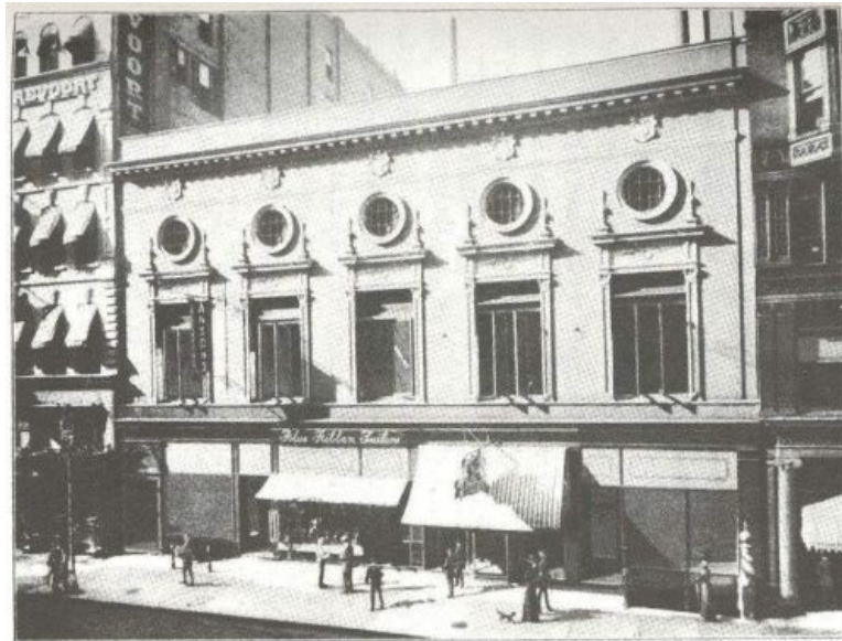
EXTERIOR OF A. C. ANSON'S BILLIARD ROOM AND BOWLING ALLEYS, CHICAGO
