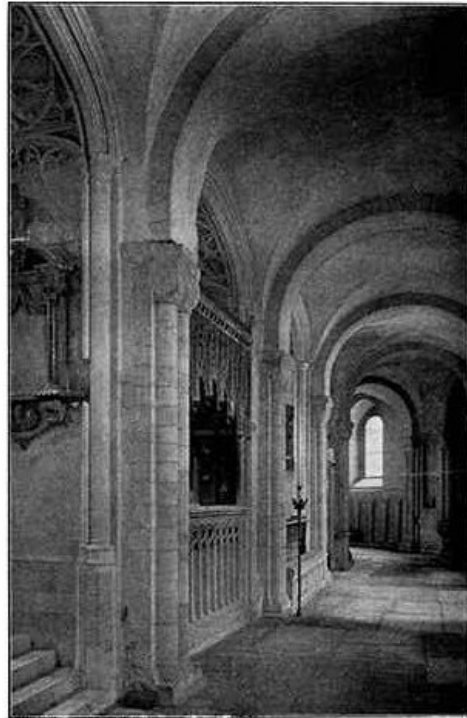
The South Aisle of Presbytery, looking East.
