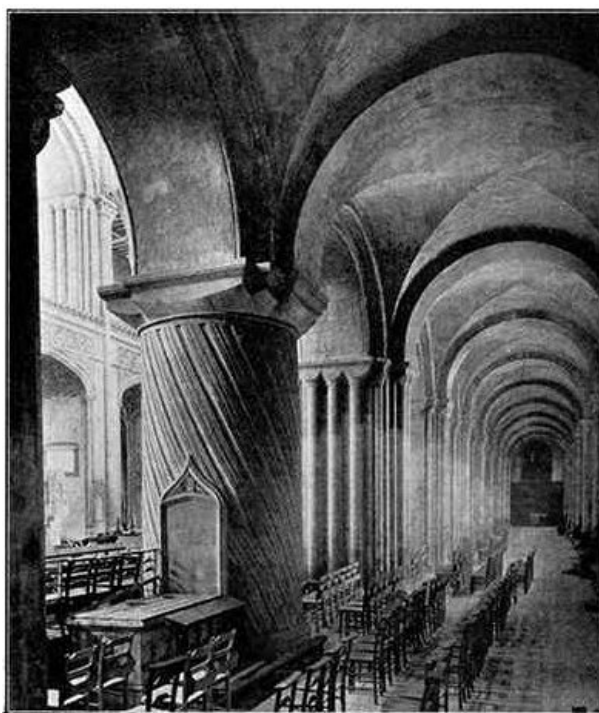
The North Aisle of Nave, looking West.
