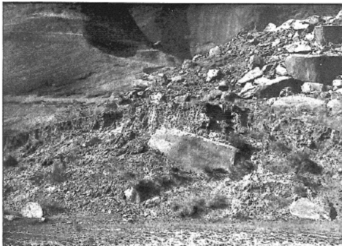
PLATE XLIV. SECTION OF OLD WALLS, CANYON DE CHELLEY
