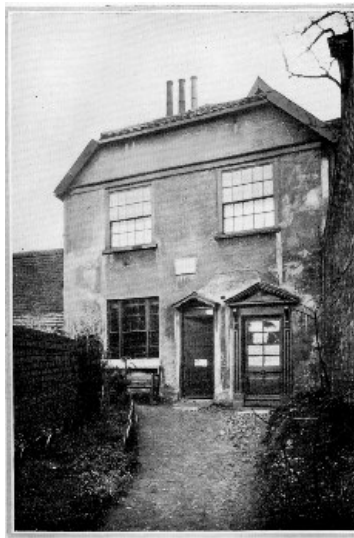
THE BORROW HOUSE, NORWICH
