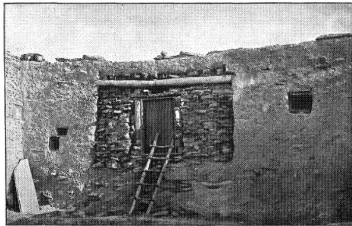
PLATE CVII. PARTIAL FILLING-IN OF A LARGE OPENING IN ORAIBI, CONVERTING IT INTO A DOORWAY.
