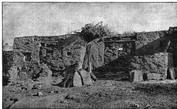
PLATE CVIII. LARGE OPENINGS REDUCED TO SMALL WINDOWS, ORAIBI.
