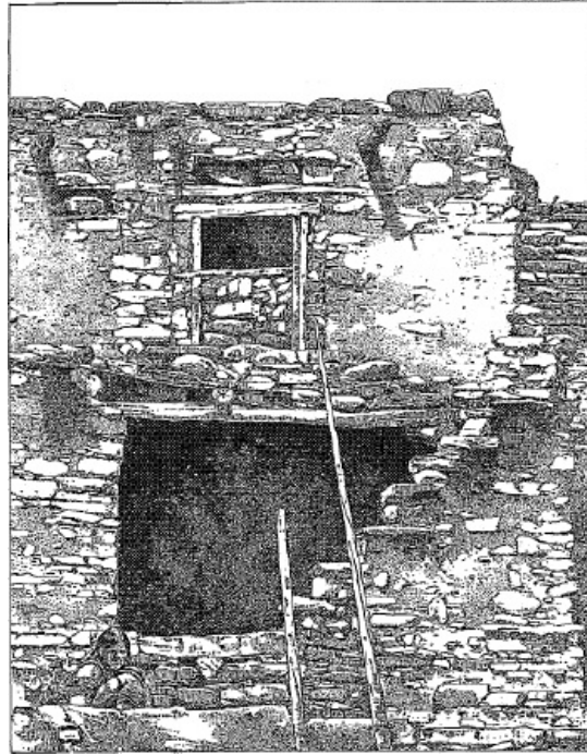
FIG. 79. Rude transoms over Tusayan openings.
