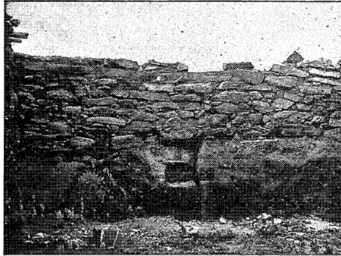
FIG. 35. An unplastered house wall in Ojo Caliente.
