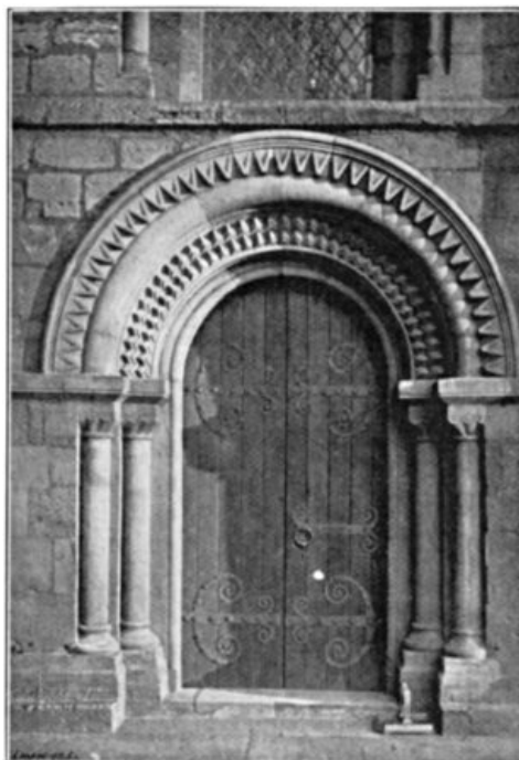
NORTH DOOR OF NAVE.
