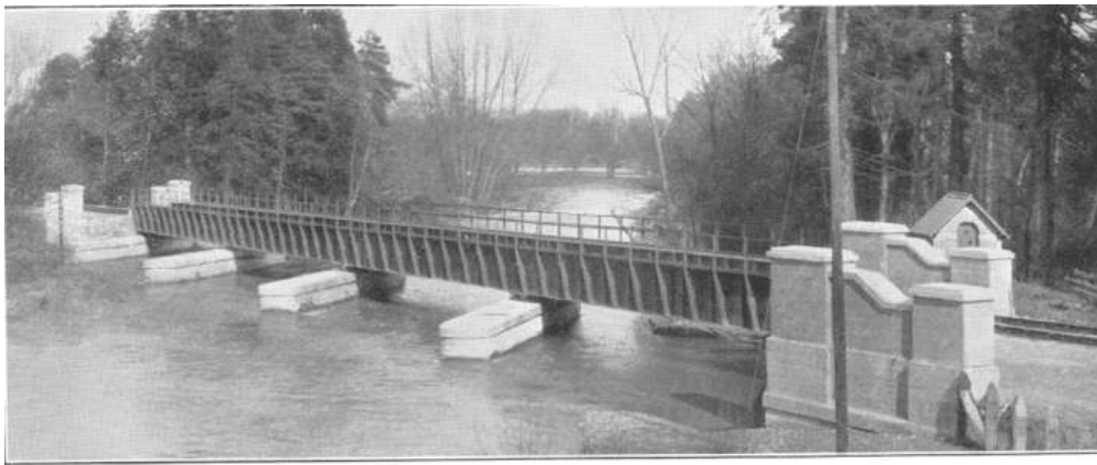
KILKEWYDD BRIDGE, near Welshpool, as recently re-built.
