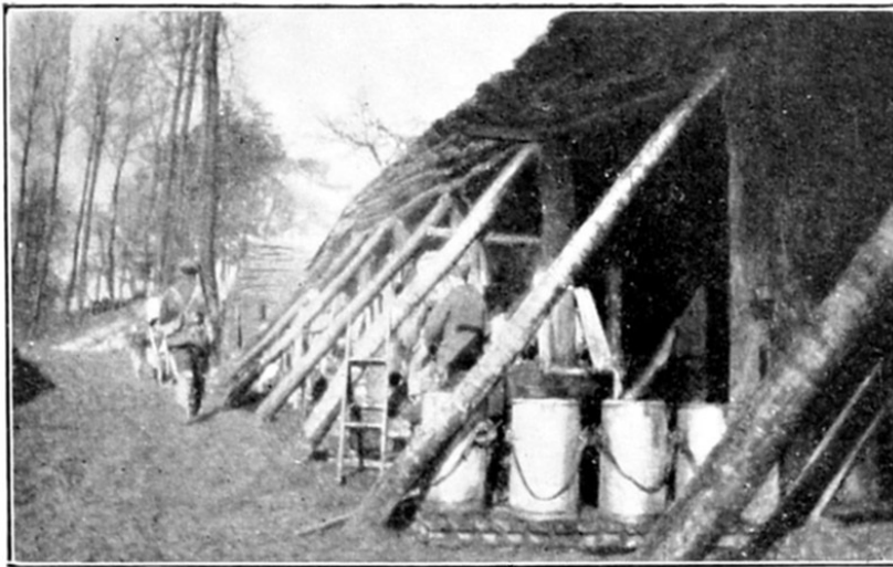
COOKHOUSE AT BECOURT.
