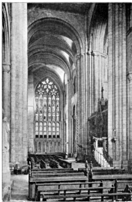
The Transepts, looking North.
