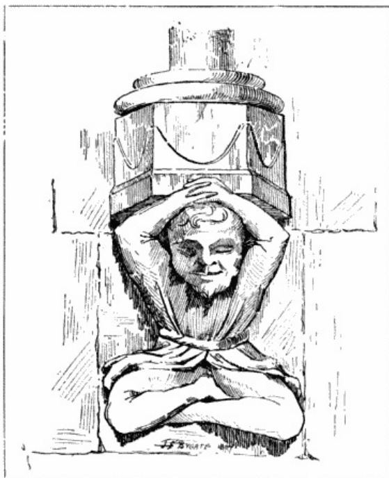
Corbel in Choir at Junction of Old and New Work.
