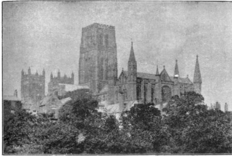
The Exterior, from the South-east.
