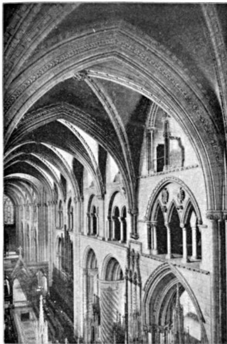
Triforium of Nave and Choir, Showing Junction of Old and New Work.
