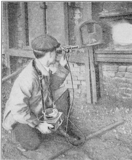
FIG. 127.—Using the optical pyrometer.
