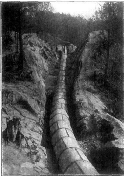
A CITY WATER SUPPLY BROUGHT FROM THE FAR HILLS
