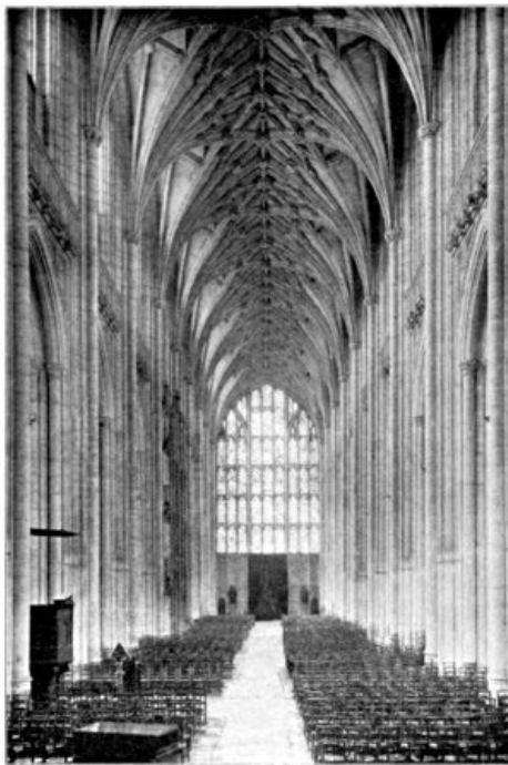
WEST WINDOW, FROM NAVE.
