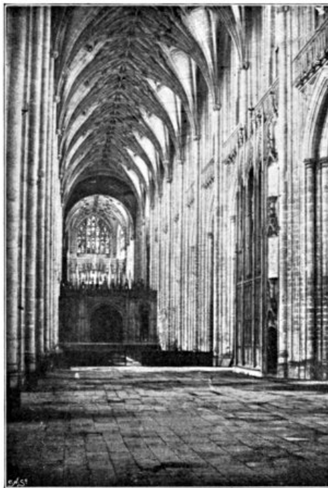
NAVE, SHOWING THE SCREEN BEFORE RESTORATION.
