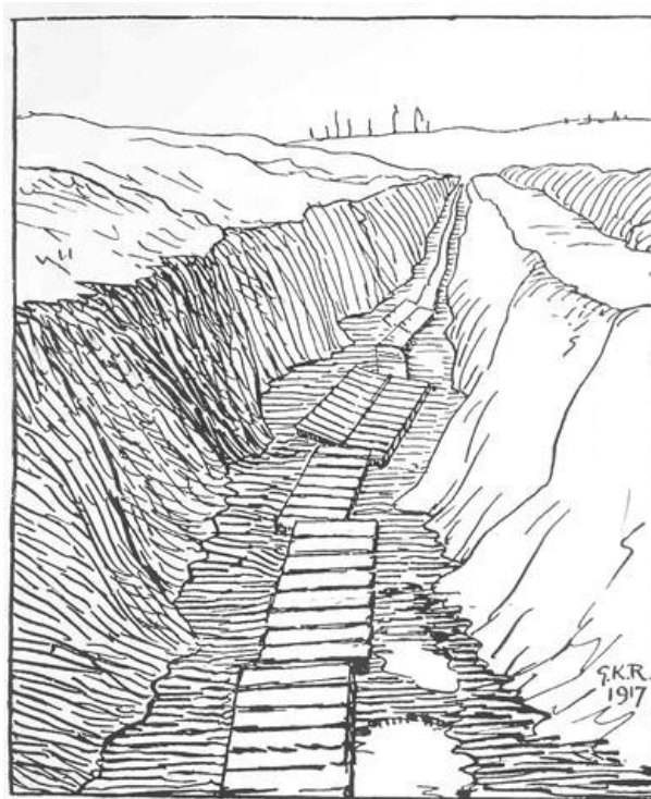
A DUCKBOARDED COMMUNICATION TRENCH
