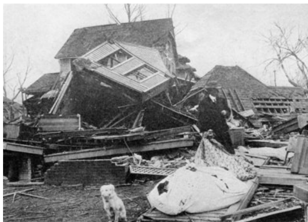
Photograph by Brown Bros. Hundreds of substantial buildings were lifted from their foundations and piled up like broken cigar boxes simply by the awful sweep of the wind
