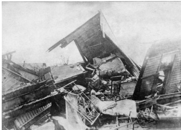
Copyright by George Grantham Bain. Hundreds of buildings were demolished by the tornado at Terre Haute, Indiana, and many lives were lost
