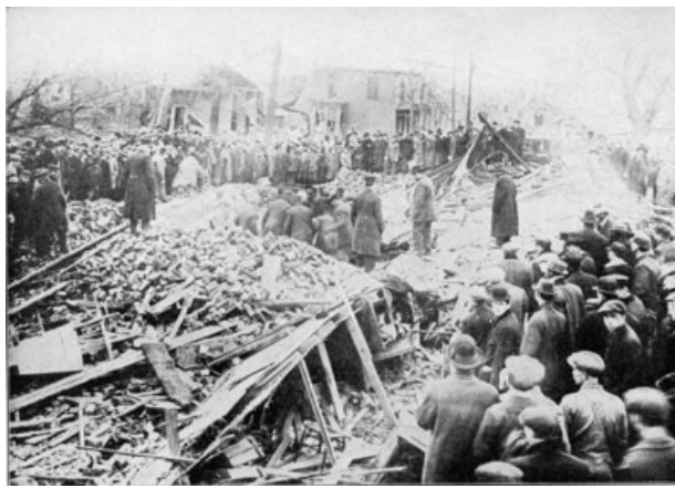
Copyright by American Press Association. Scene showing a section of Omaha entirely wrecked. On the left is all that remains of Idlewild Hall. At this spot a large number of people were killed
