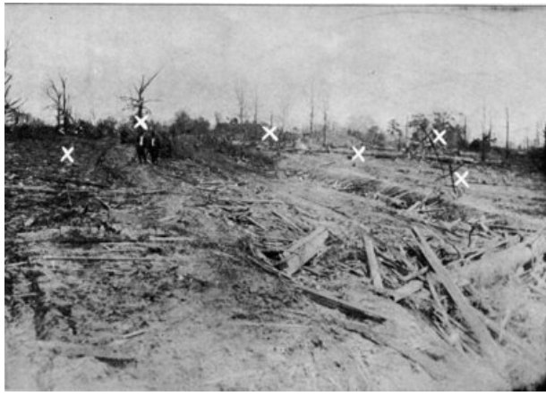
Copyright by Underwood & Underwood, N. Y. Showing what was once the town of Lower Peachtree. The six X's denote the places where houses stood before the tornado, in the heart of the main residential streets
