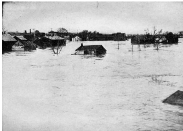
Copyright by Underwood & Underwood, N. Y. The flood at Watervliet, New York, showing buildings torn from their foundations and floating down the stream. Great damage and untold suffering resulted
