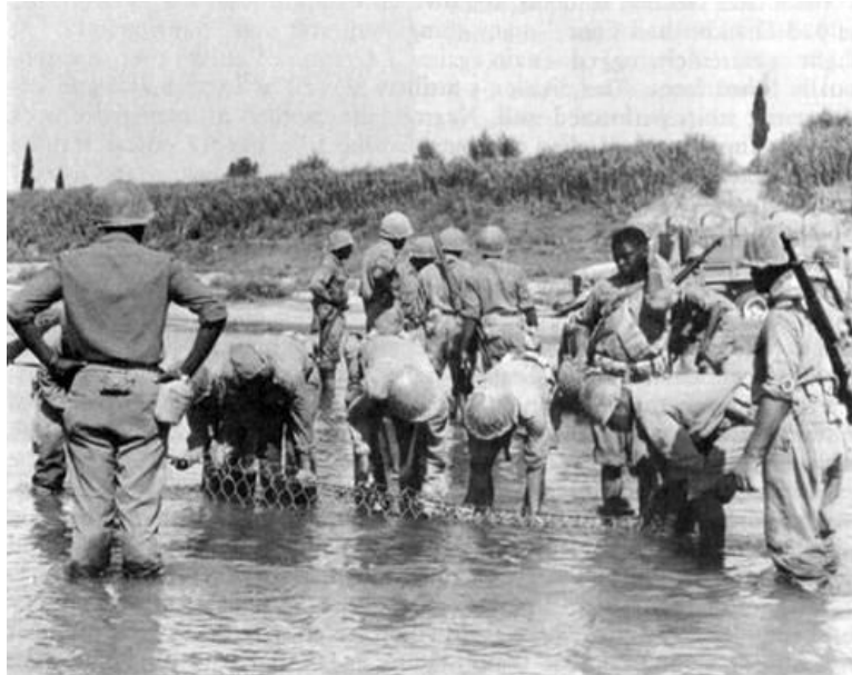
92D DIVISION ENGINEERS PREPARE A FORD FOR ARNO RIVER TRAFFIC
