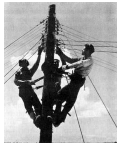
ELECTRICIAN MATES string power lines in the Central Pacific.
