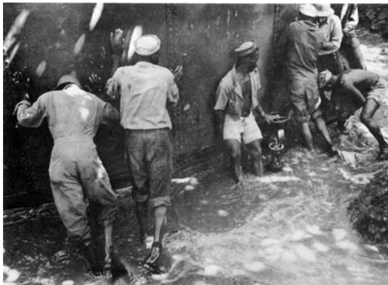
SEABEES IN THE SOUTH PACIFIC righting an undermined water tank.
