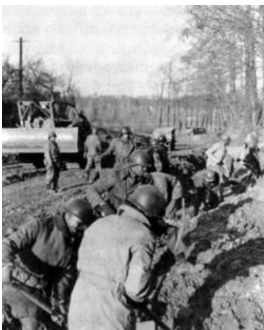
ROAD REPAIRMEN, Company A, 279th Engineer Battalion, near Rimberg, Germany, December 1944.
