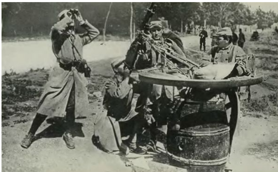
French Using an Ordinary Wine Barrel on which a Wagon Wheel Is Mounted to Facilitate the Revolving Movement to Any Desired Direction.
