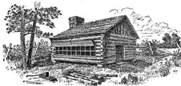
FIG. 292. AN UNIMPROVED SCHOOLHOUSE
