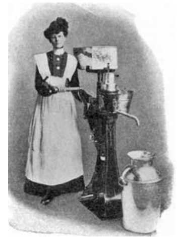
FIG. 271. A HAND SEPARATOR
