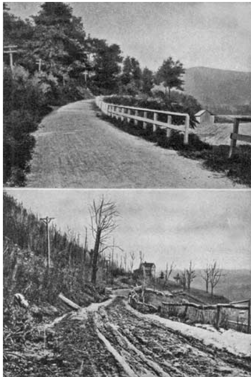
FIG. 294. THE SAME ROAD AFTER AND BEFORE IMPROVEMENT
