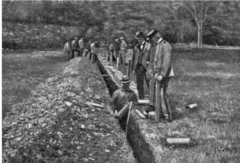
FIG. 9. LAYING A TILE DRAIN
