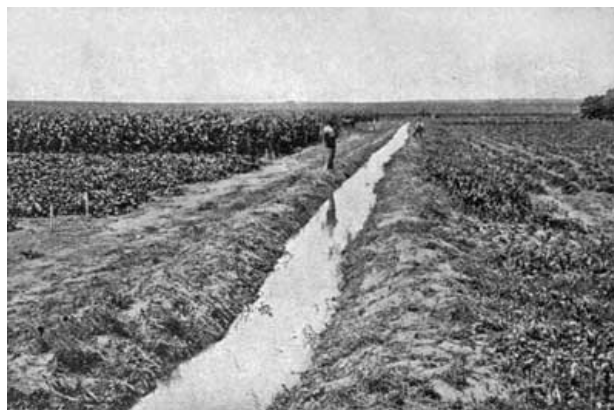
FIG. 287. THE MAIN DITCH OF AN IRRIGATION PLANT
