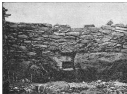
FIG. 35. An unplastered house wall in Ojo Caliente.
