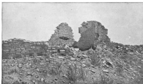
PLATE LXV. STANDING WALLS OF KIN-TIEL.
