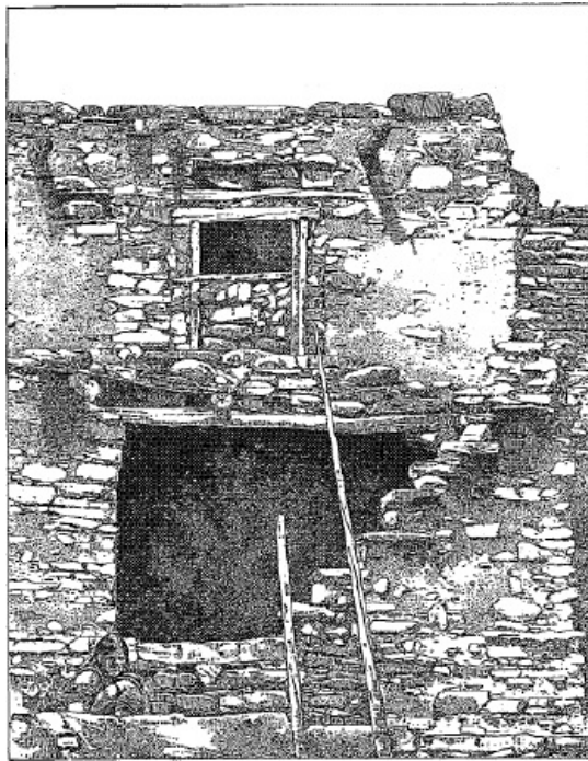
FIG. 79. Rude transoms over Tusayan openings.
