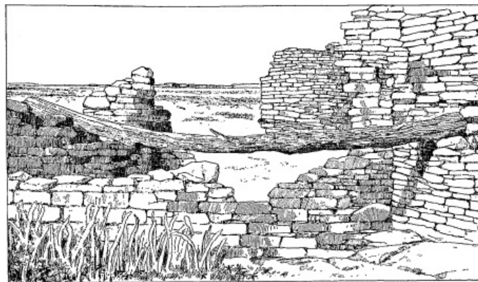
PLATE XCV. ANCIENT FLOOR-BEAMS AT KIN-TIEL.
