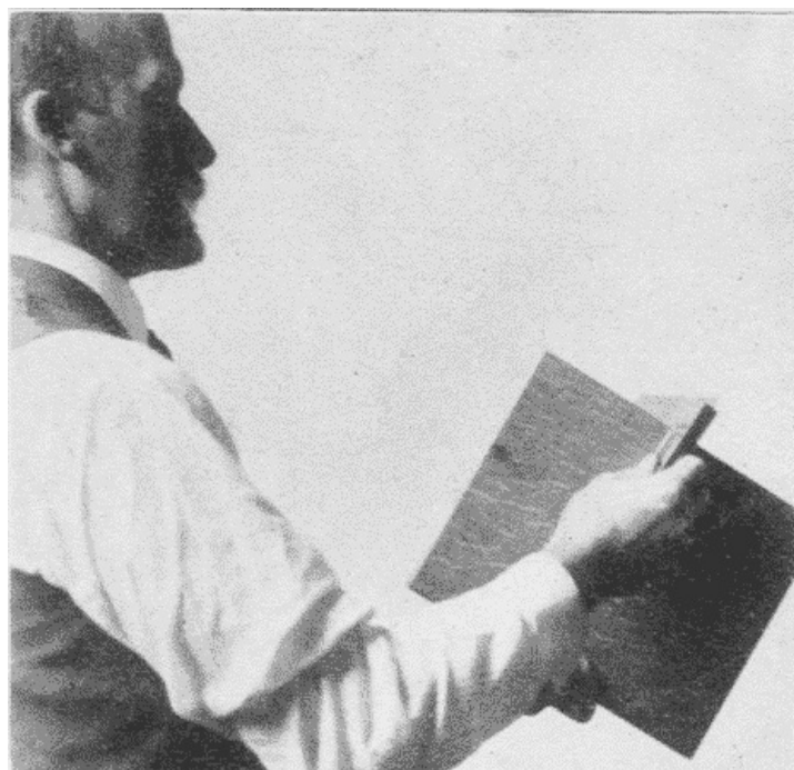
Fig. 203. Using the Try-Square.
