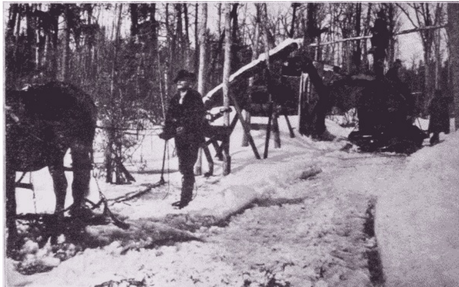
Fig. 10. Making an Ice Road by Flooding.
