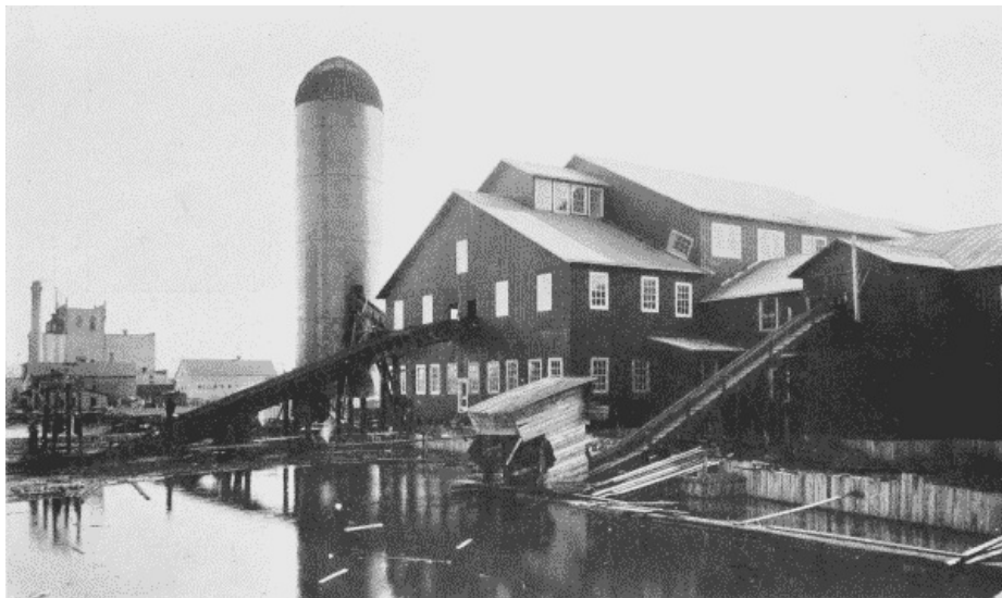
Fig. 37. Two-Story Mill at Virginia, Minnesota, Showing Jack-Ladders and Consumer.
