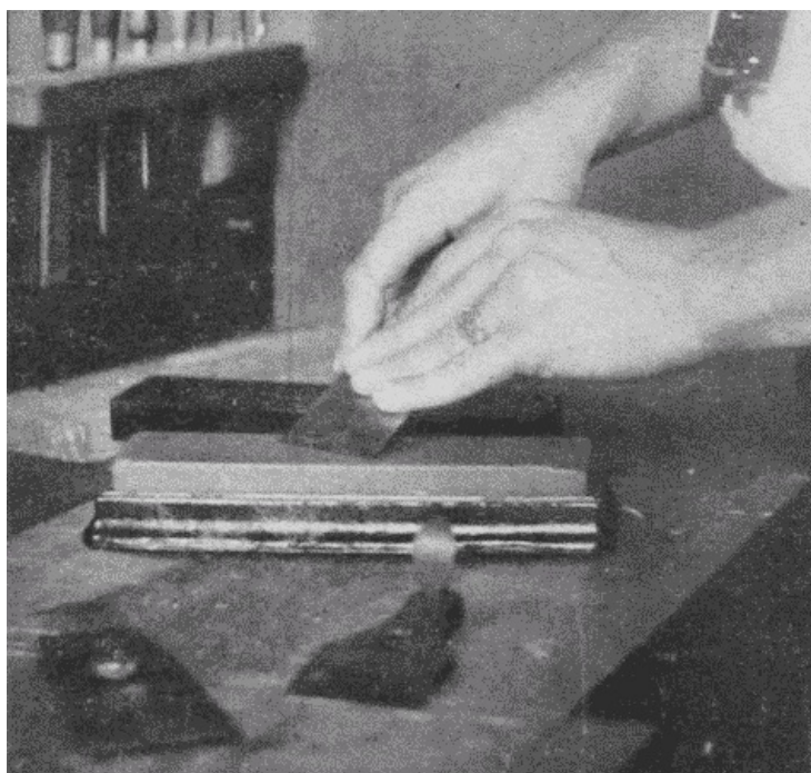
Fig. 77 Whetting a Plane-Bit.
