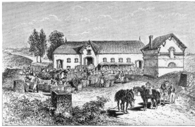
THE ESTABLISHMENT OF MESSRS. CHARLES FARRE & CO., AT HAUTVILLERS. (p. 15)
