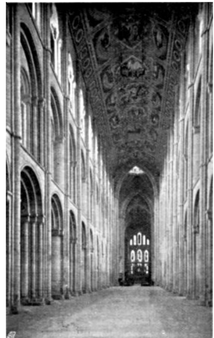
THE NAVE, LOOKING EAST.
