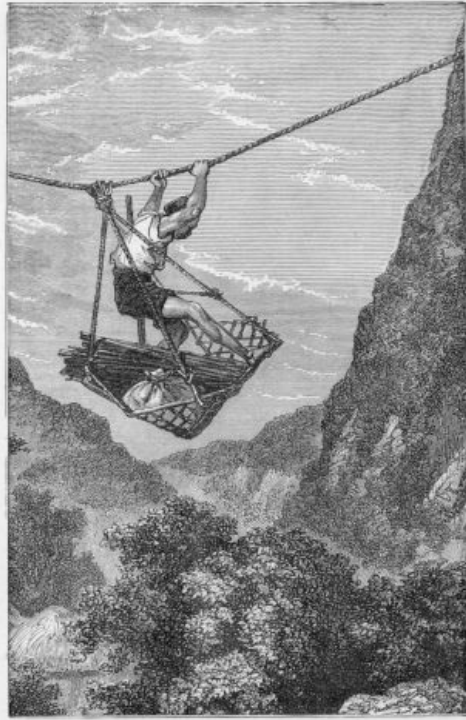
CROSSING A ROPE-BRIDGE.
