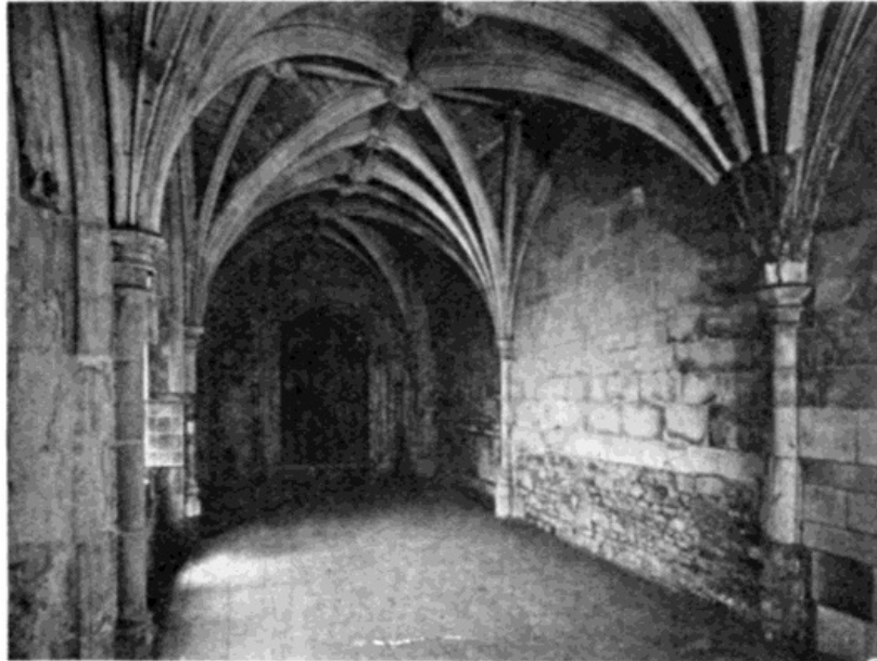
THE REMAINING BAYS OF THE CLOISTER
