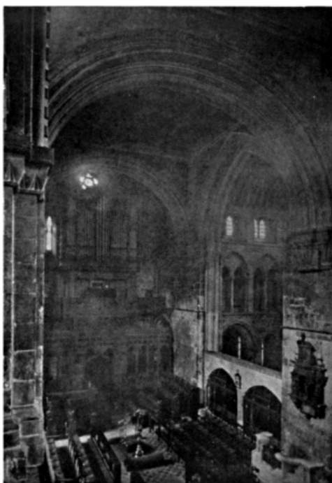
VIEW OF THE CROSSING FROM THE TRIFORIUM
