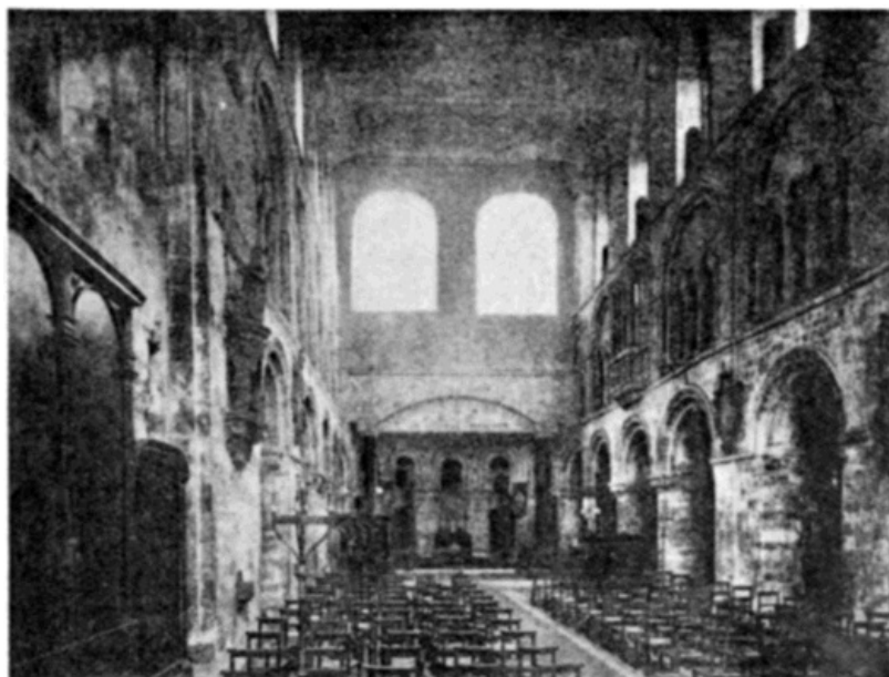
THE CHOIR BEFORE RESTORATION, SHOWING THE FACTORY FLOOR EXTENDING OVER THE APSE AND SUPPORTED BY TWO IRON COLUMNS
