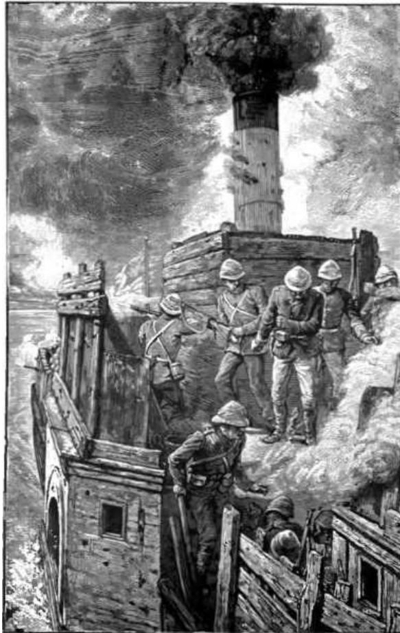
"A SHOT HAD PASSED THROUGH HER BOILER."
