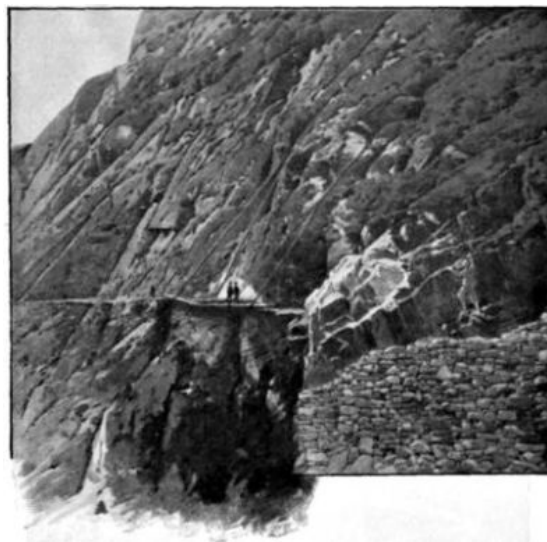
A SHAKY PASSAGE ON THE NERPANI ROAD
