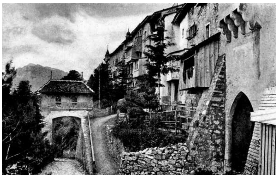
FORTIFIED HOUSES—NORTH WALL
