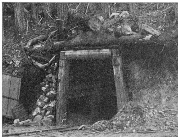
FIG. 98.—MOUTH OF A TUNNEL
