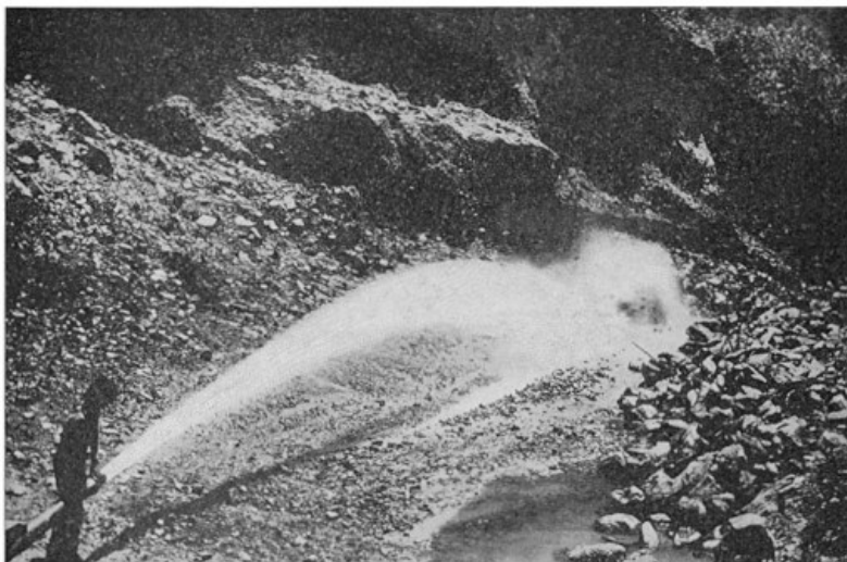
FIG. 100.—HYDRAULIC MINING ON THE KLAMATH RIVER, CALIFORNIA
