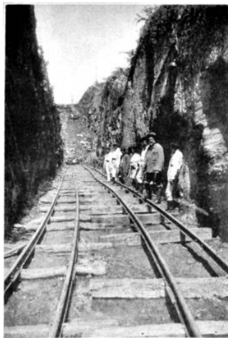
GOYAZ RAILWAY IN CONSTRUCTION. The cut leading to the Paranyhyba River.
