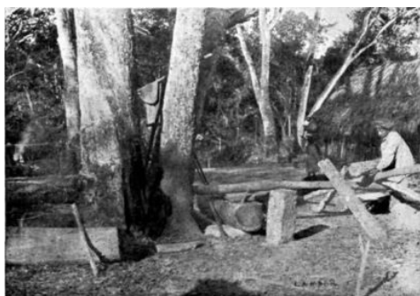
METHOD OF PRESSING RUBBER INTO CAKES. The alum process of coagulation being used.
