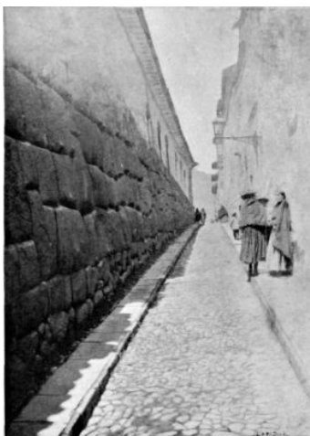
A FAMOUS INCA WALL, CUZCO. The various rocks fit so perfectly that no mortar was used to keep them in place.
