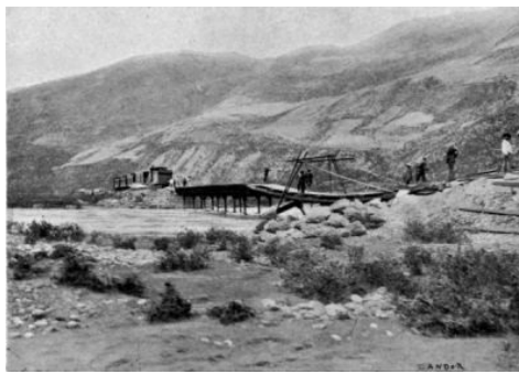
ON THE WAY TO CUZCO. Railway bridges partly carried away by swollen river.
