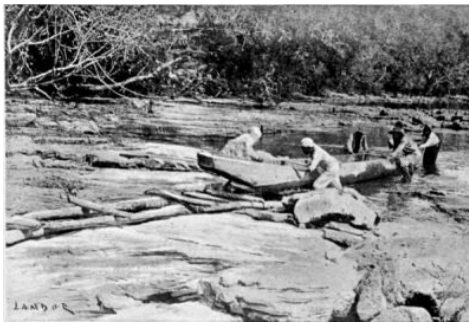
THE WOODEN RAILWAY CONSTRUCTED BY AUTHOR IN ORDER TO TAKE THE CANOE OVERLAND FOR TWO AND A HALF KILOMETRES AT THE AUGUST FALLS.
