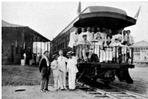
THE INAUGURATION TRAIN ON THE MADEIRA-MAMORE RAILWAY.
