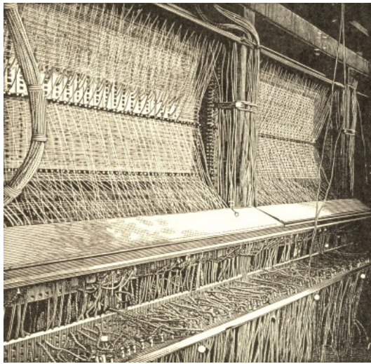
Under Side of a Modern Switchboard, showing 2,000 Telegraph Wires.
