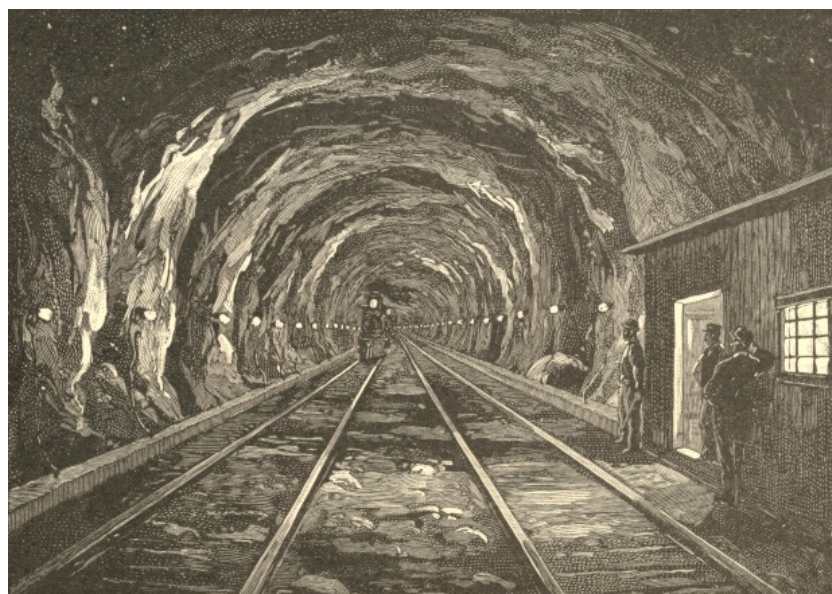
The Hoosac Tunnel Lit by Glow Lamps, after the Plan of the Marr Construction Company.
