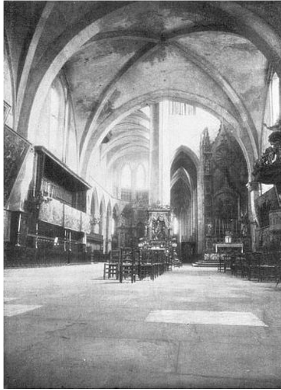
"THE NAVE OF THE XIII CENTURY IS AN AISLE-LESS CHAMBER, LOW AND BROADLY ARCHED."—TOULOUSE. [To List]
