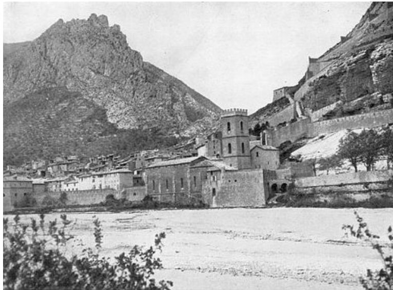
“THE CHURCH TOWER STOOD OUT AGAINST THE ROCKY PEAKS.”—ENTREVAUX. [To List]
