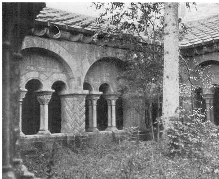
"THE GREAT PIERS AND SMALL FIRM COLUMNS."—VAISON. [To List]
