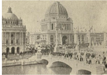
The Administration Building, seen from the Agricultural Building.
