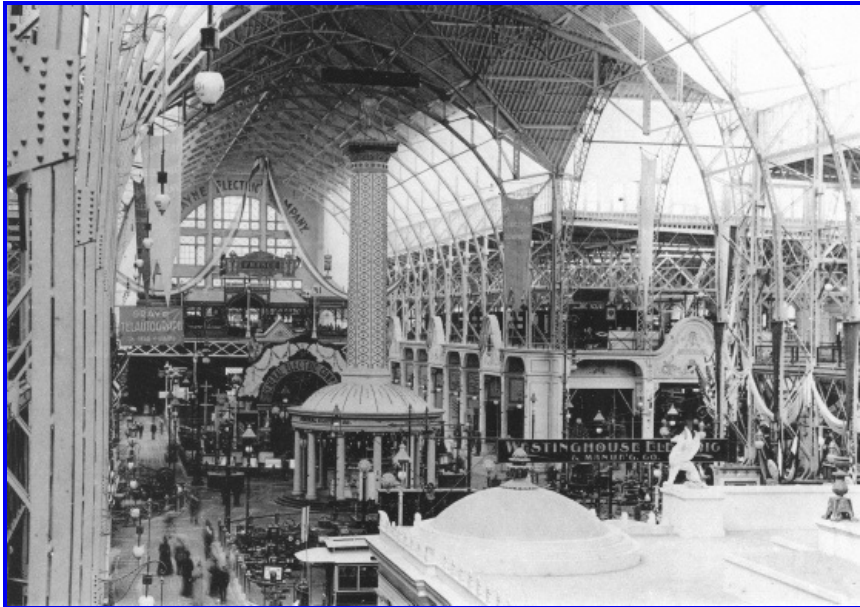
PLATE 30--INTERIOR OF ELECTRICITY BUILDING.
