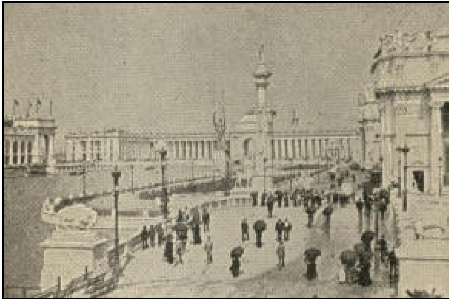
A view toward the Peristyle from Machinery Hall.
