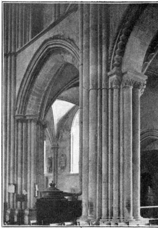
JUNCTION OF NORMAN AND EARLY ENGLISH WORK, ON THE NORTH SIDE OF THE NAVE
