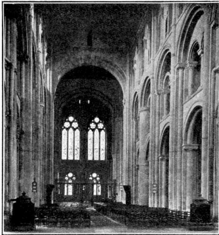
THE INTERIOR FROM THE WEST
