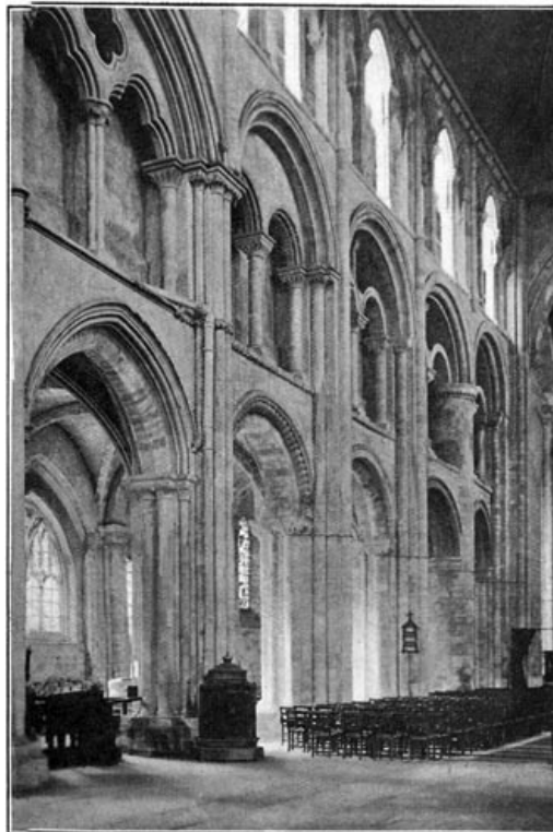
THE NAVE, NORTH SIDE
