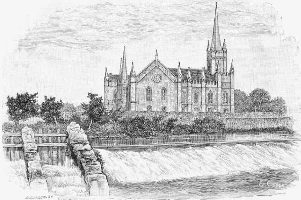
ROMAN CATHOLIC CHURCH AT PARSONSTOWN.
